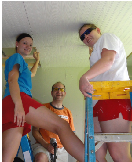
Installing the ceiling panels in bunk rooms
