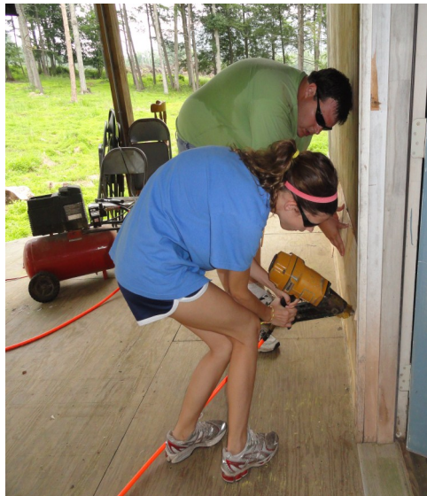
Siding the Amphitheater building
